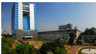
Figure 1.4 Main Building of Ministry PUPR - Jakarta Source: PUPR Ministry (2023)
