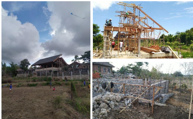
Figure 3 : CLC during Construction (Author's Documentations, 2019)
